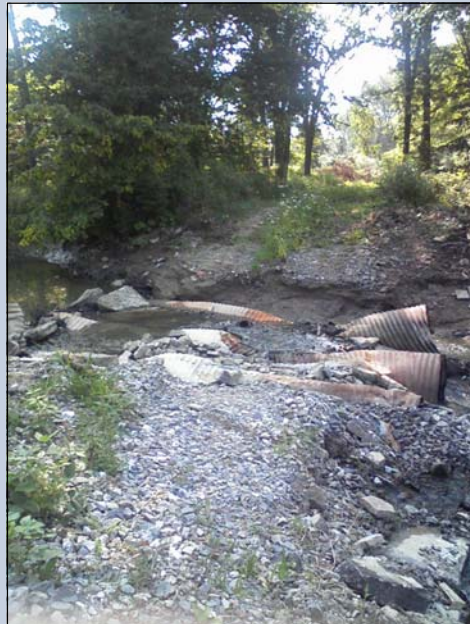
Fish Barrier #103 - Currently in progress
